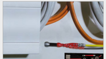
Shafts and underfloor ducting
